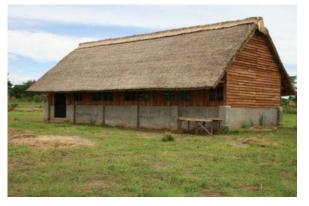
**13 Administration 1.** Finished covering, cross ventilation, assembled and fixed window frames(↑).
