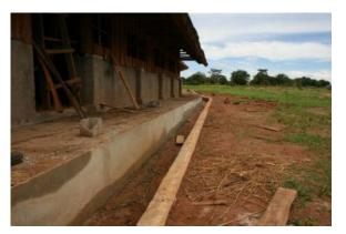
**Veranda.** On the girl's wing, on the front side of the veranda we finished the gutter except for filling it with crushed stones( $\uparrow$ ). At the back we finished digging and putting PVC and deformed bars( $\downarrow$ ).
